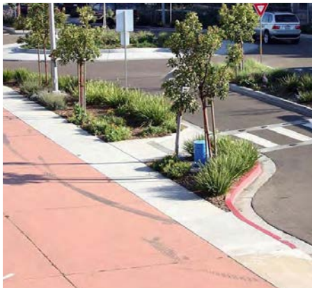
Coloured concrete in median paving area.
