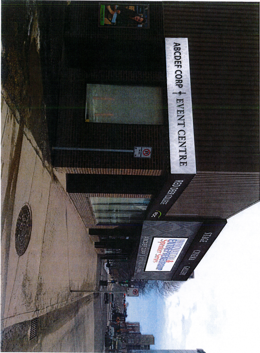
West Side > Non-illuminated dimensional letters on panel with original cinema graphic style background > Refinished corrugated metal paneling
