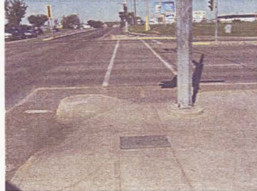
Steel plate near ramp a trip / slip hazard
