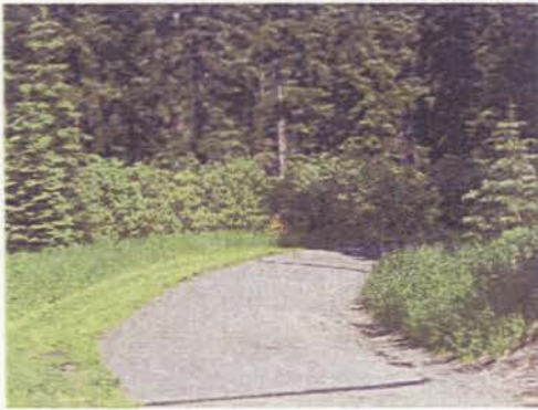
Steep slope with blind corner, near McKenzie Trail. Widening trail, creating a centerline, and clearing would improve this situation.
