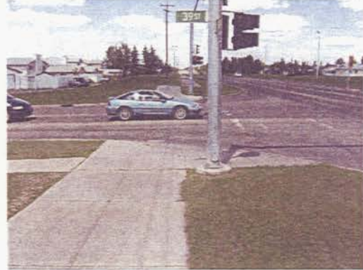
Trail alignment behind stop bar. Pedestrian crossing in bad location. 30 th Ave. & 39 th St.
