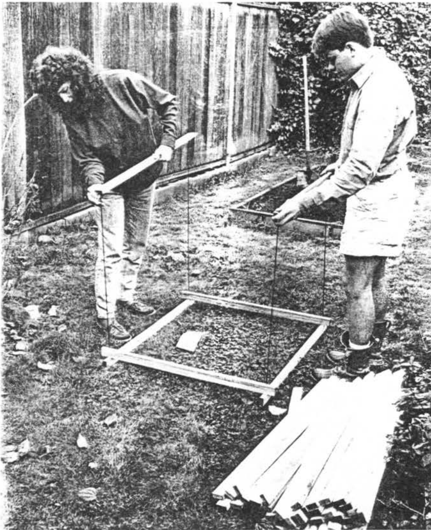
The easy-to-assemble composting bins used in the King County project are constructed of alternating cedar slats with four metal connector rods. Residents participating in the project receive information from the county on how to compost their yard wastes.
