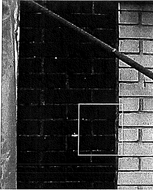
Construction Photo showing mortar damage from stone veneer anchors and high pressure washing
