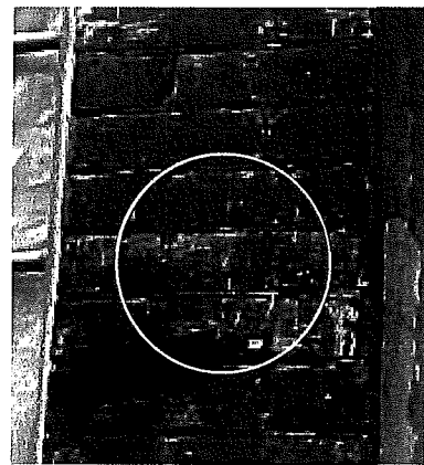
Construction Photo showing original coloured, beaded mortar joints as well as damage from stone anchors, pressure washing. Brick damage is from unknown source.
